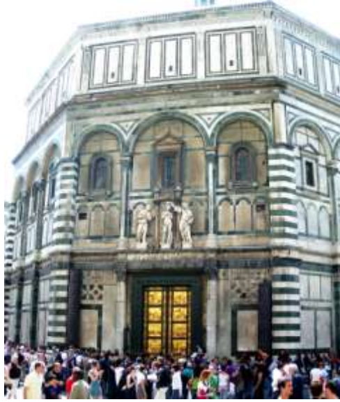
The baptistry showing the gold door and the upper floors.
