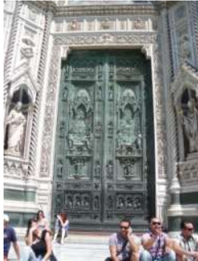
Detail of the front door .
