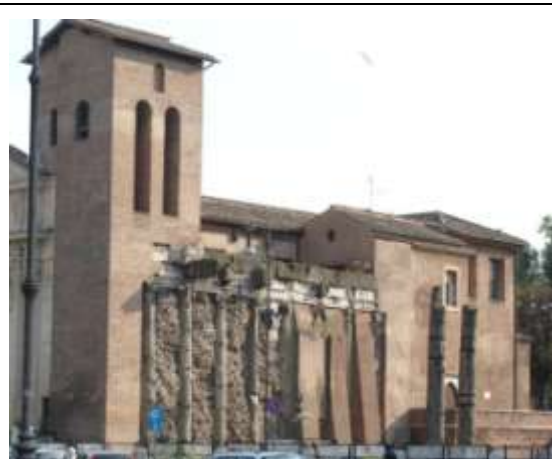
This is a working church that has preserved four ancient columns and part of a wall into a newer bell tower.
