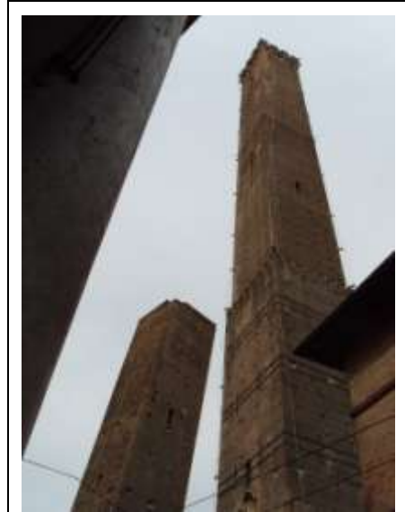
Due Torri . The short one leans more than the tower at Pisa.
