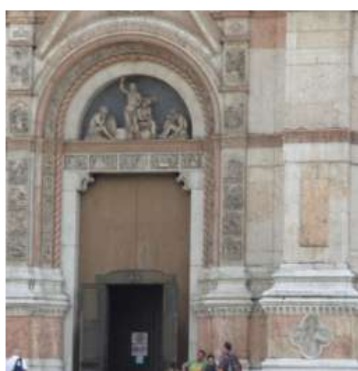
The finished part of the Basilica's façade has white and pink marble.
