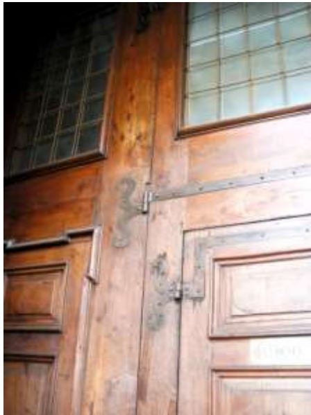
Very old handmade doors & hinges are still in use.
